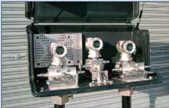
IEX3 Enclosure with heating system
